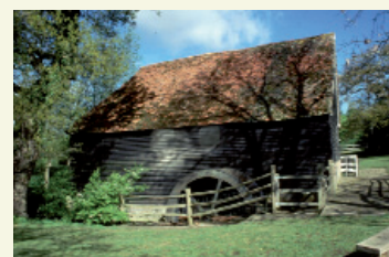
The restored Watermill at Michelham Priory
