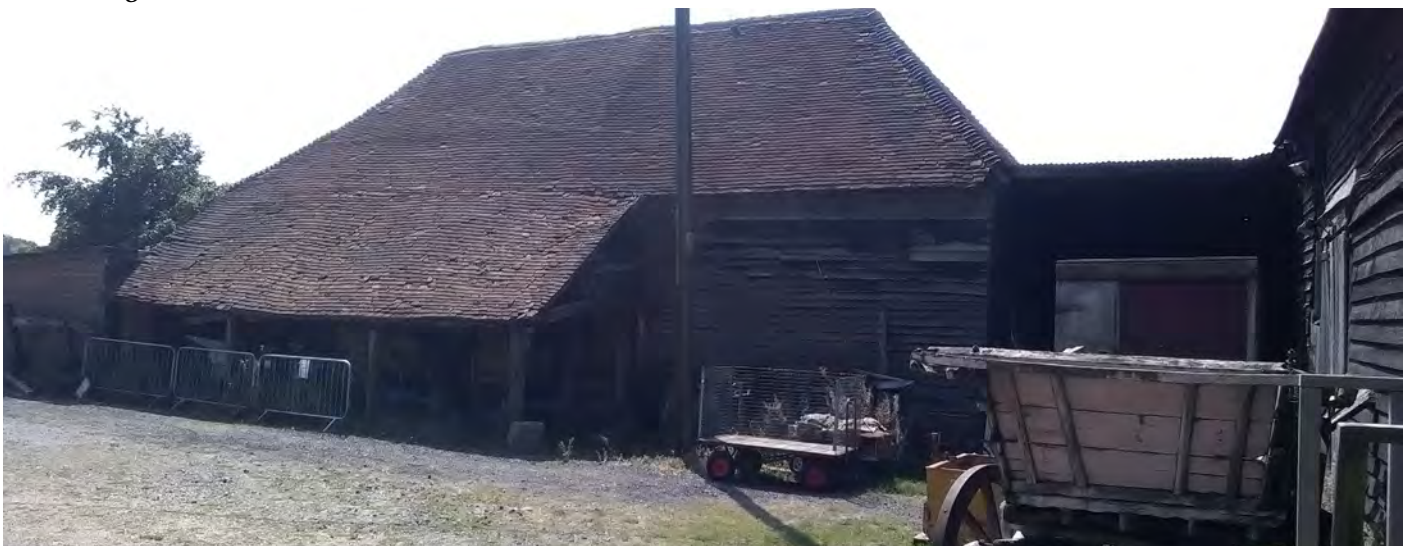
Typical View into Site
